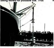
Engineers watch front mounted hydraulic pole digger in operation
