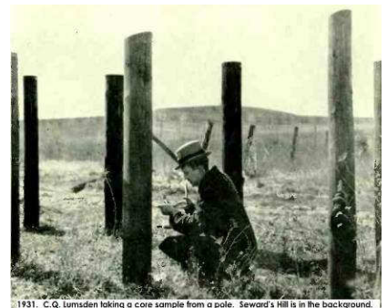
1931. C. Q. Lumsden taking a core sample from a pole. Seward's Hill is in the background.
