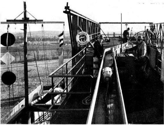
Engineers study section of cable containing dummy amplifier being played out. Inscription on life preserver stands for "Bell Laboratories Dry Land Cable Ship Fantastic."
