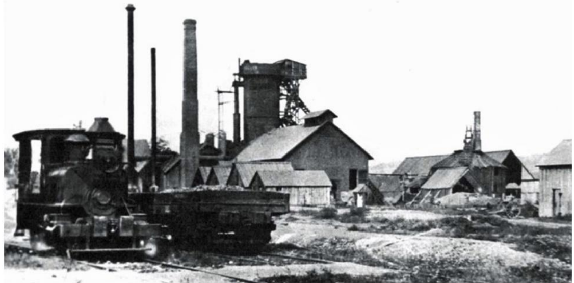
The only known picture of William J. Taylor's Chester Furnace. A locomotive used to move cars around the site is shown. The 60' tall blast furnace stack is center. A spur of the CNJ Chester Branch serviced the site.
