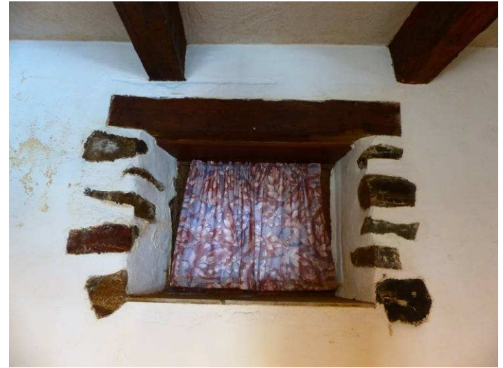
Window on northeast side of the barn
