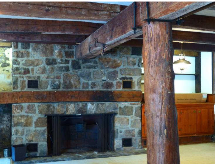
Basement fireplace, trunk supports, and beams
