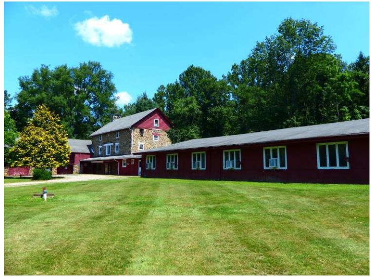
Southwest view of the barn and convalescent wing
