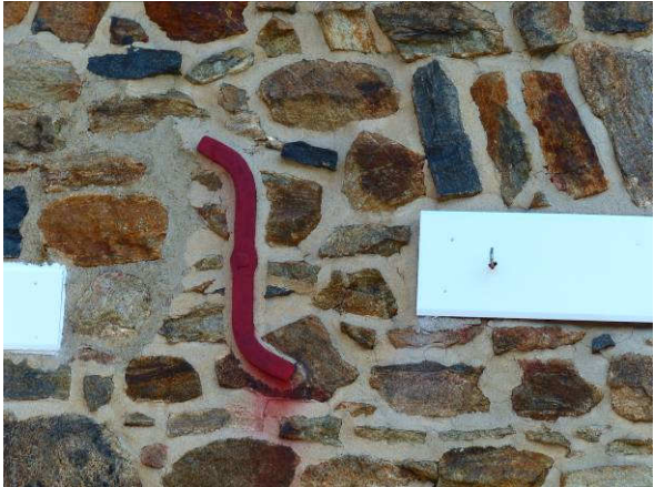
Enlarged view of S anchoring iron
