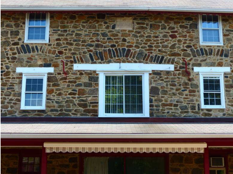
Windows, arches, datestone, and S anchoring irons.
