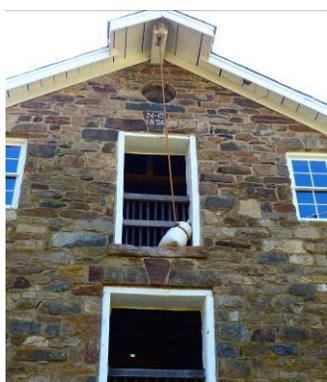
Grain is hoisted to & cleaned on 3rd floor
