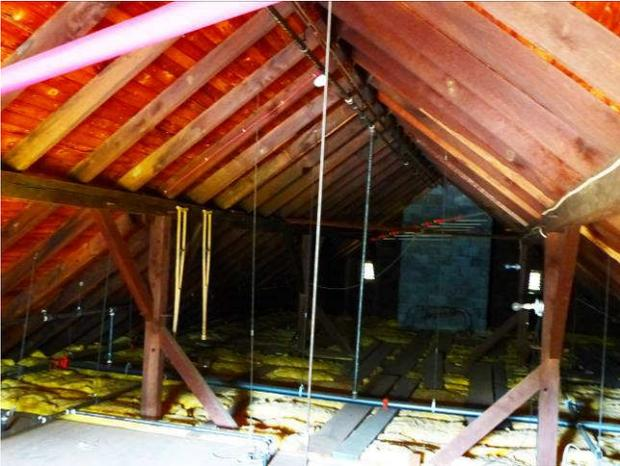
Left: image of the attic. New roof and rafters replaced the original. The vertical support beams are original.
